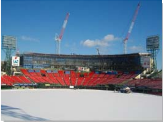
Facilities around Backstop
